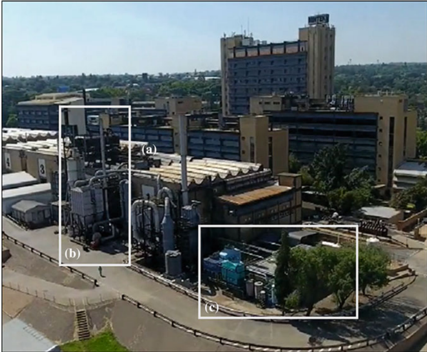
Fig. 9 Aerial view of the bays and office blocks at Mintek from the North-Western side of campus. Bay 2 (a), the off-gas cleaning plant for Bay 2 (b), and the water-cooling plant for all of the pilot-scale facilities (c) are indicated
